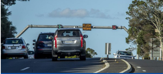
Dynamic lanes, such as those used on Whangaparāoa Rd, use the flush median to open up more lanes for traffic during peak hours.
