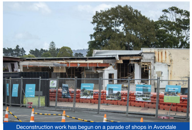
Deconstruction work has begun on a parade of shops in Avondale
