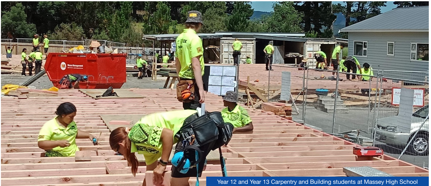
Year 12 and Year 13 Carpentry and Building students at Massey High School
