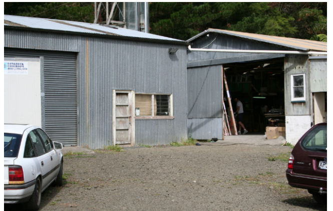
Above: 1997 C-Tech's operation was housed in the above shed. Below: The 2010 construction of C-Tech's current headquarters.
